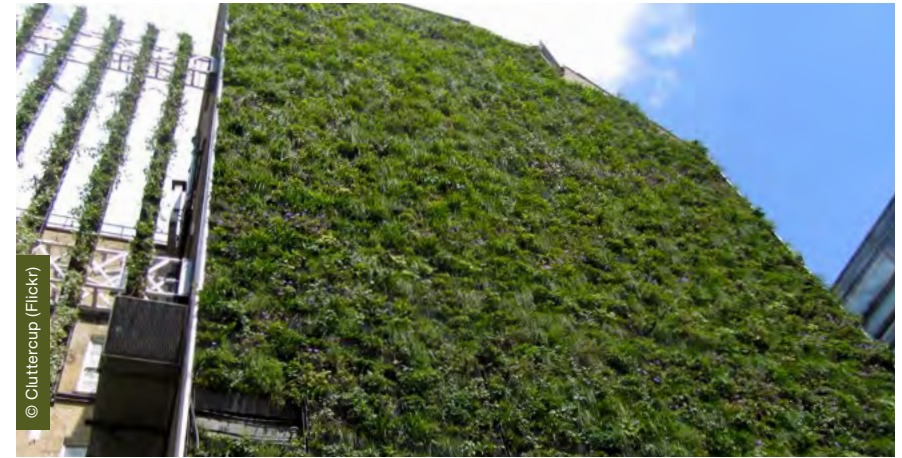
Green Wall, The Palace Hotel, London: Living walls can make a significant contribution to building cooling and insulation, thereby helping to lower energy consumption.
